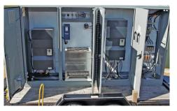
**MOTOR CONTROL PANEL.** The motor control panel provides options to configure a control system that best fits your application – whether that's a soft-start or VFD panel.
