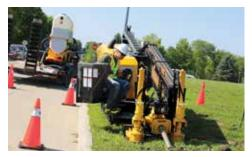
**RIGHT POWER, RIGHT FOOTPRINT.** The D20x22 S3 offers a sizeable increase in power and rotational torque over its predecessor, the D16x20 Series II, making it well-suited to install cable, fiber and product pipe efficiently and productively.
